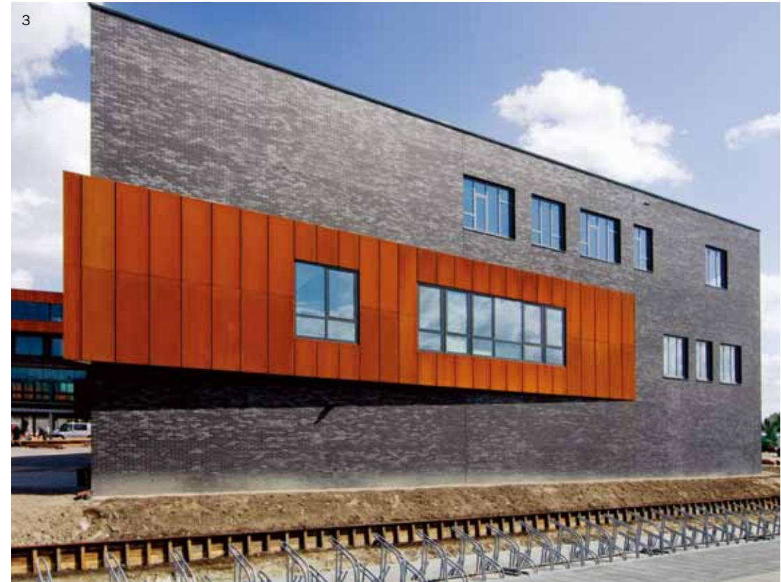
1. Overall view of water bank building 2, 3, 4. Contrasting colours and materials are also used on the exterior; dark brick façades are clad with corten steel
