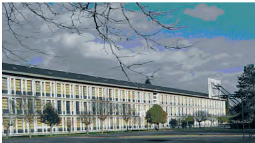
Figure 1.11 REVIVAL building Lycée Chevrolier, Angers, France: Built in 1958 of pre-cast concrete construction with dry lining and poorly fitting metal windows, it had very high infiltration rates before refurbishment
