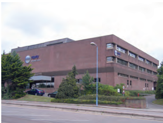
Figure 1.5 Deep-plan buildings such as these, built in the era of cheap energy and relying on air-conditioning and artificial lighting, may present insurmountable problems for sustainable refurbishment
