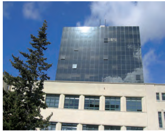
Figure 1.9 An over-glazed lightweight building of the 1970s suffering from overheating in summer and under-heating in winter. The client's perception is often that the only solution to comfort problems is air-conditioning
