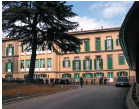
Figure 1.6 REVIVAL building Meyer Hospital, Florence: Refurbishment accompanies change of use from nursing area to hospital administrative and reception area, involving different environmental conditions
