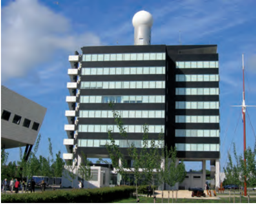
Figure 1.7 REVIVAL building The Albatros, Den Helder, The Netherlands: Refurbished in conjunction with change of use from residential to offices
