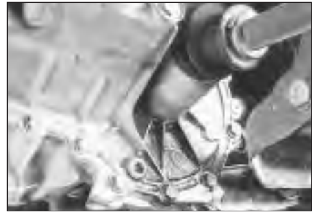
Gearbox oil can leak from the seals at the inboard ends of the driveshafts.
