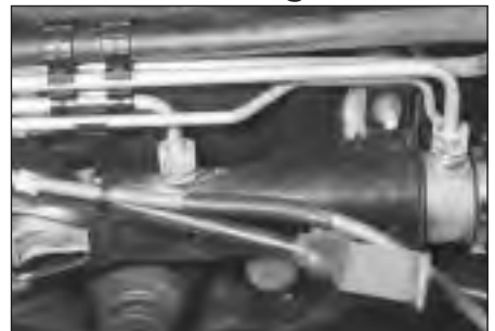
Power steering fluid may leak from the pipe connectors on the steering rack.
