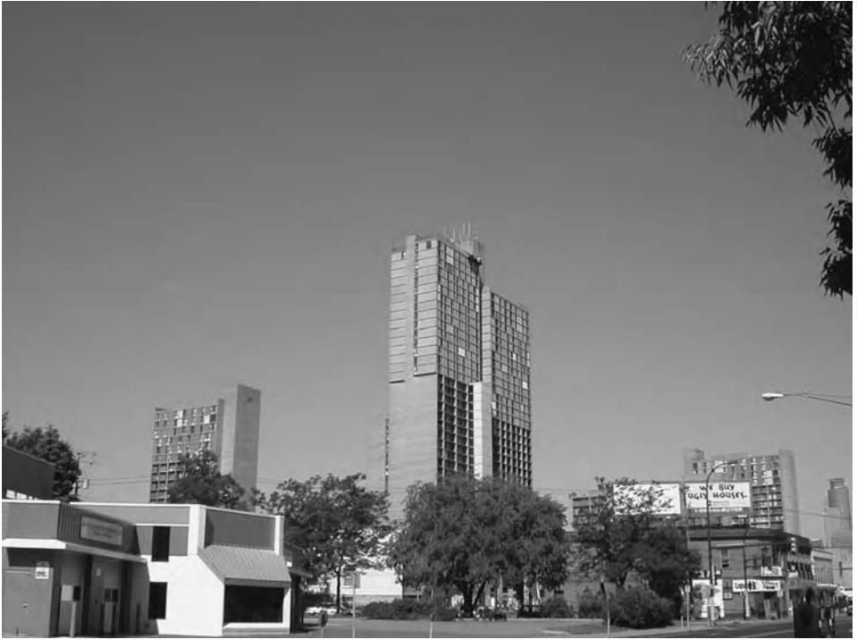
Plate 7.3 Not so aesthetic for creative people: Riverside Plaza in Minneapolis, Minnesota
