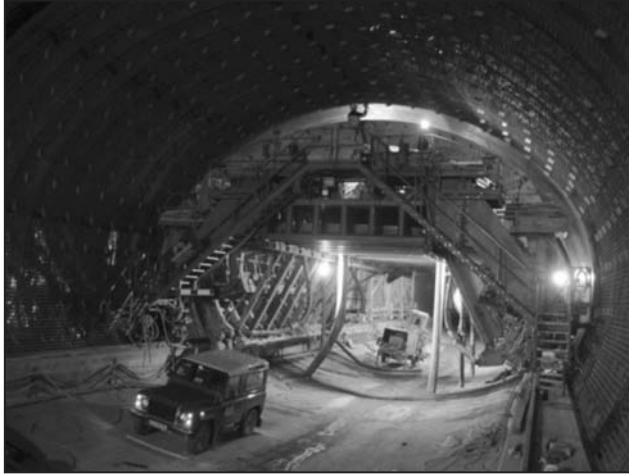
Figure 2.8 European-style form for NATM tunnel
