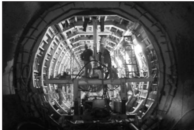
Figure 2.4 Telescopic formwork—expanded full-round tunnel form with concrete injector in place
