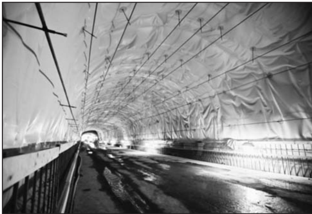
Figure 2.6 Waterproofing membrane in place with sealed dowels to support template bars
